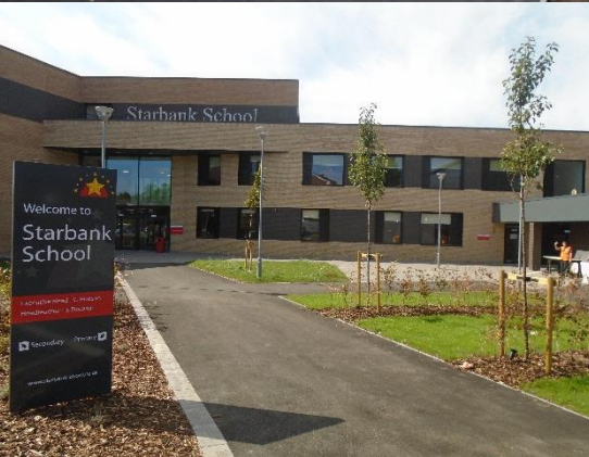
Starbank All-through School, Birmingham
